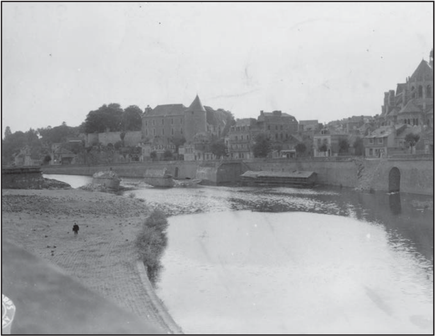
One of the destroyed bridges in Mayenne, south of the bridge seized by the 1st Battalion, 357th Infantry.
